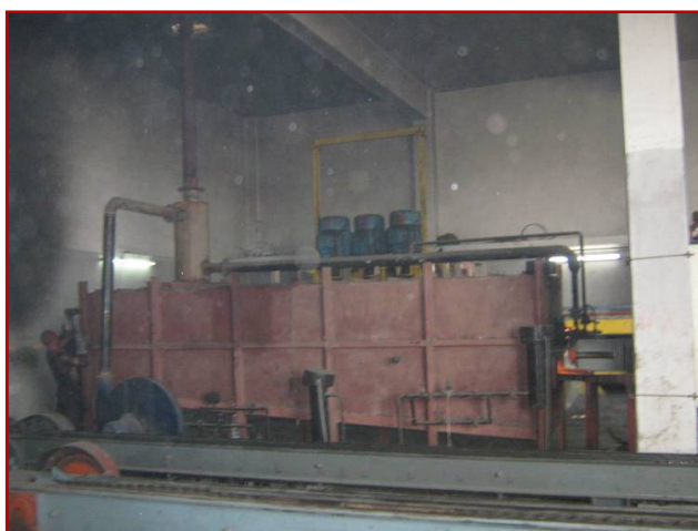
Figure2.1: Energy efficient reheating furnace
